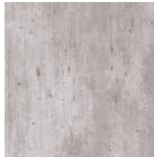
2204 S Cracked Cement Grout line none
